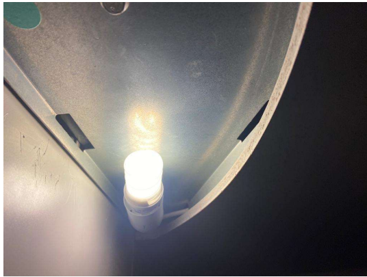
Light fitting with Edison lamp holder and bulb
